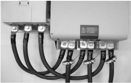
Figure 9.15 - CTs to external current aquisition
